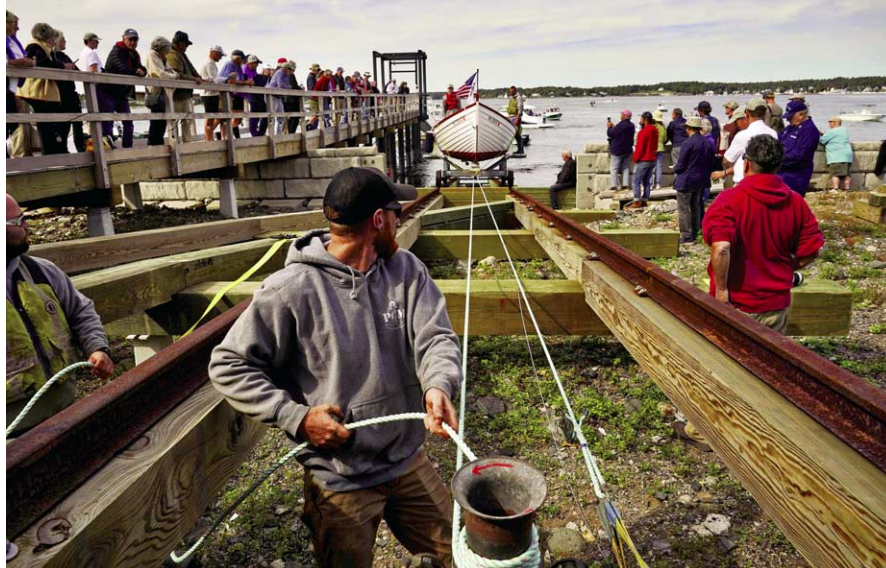
The restored 200-foot marine railway at Wood Island is the only one in the country still connecting a life saving station to the water.
